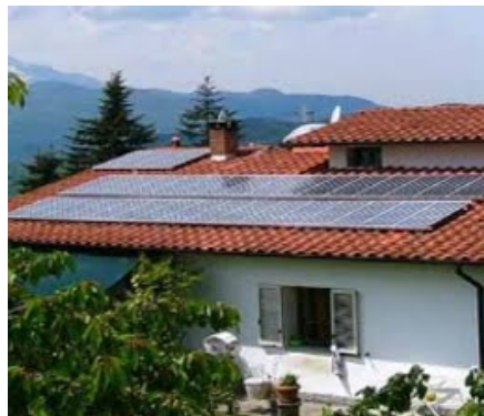
Figure 1: An installation of photovoltaic panels
